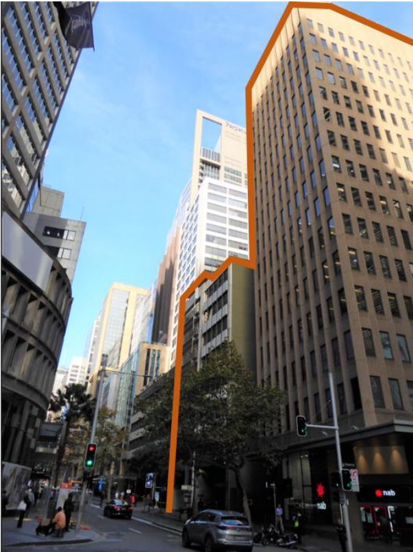
Figure 3: Subject site on the corner of Hunter and Pitt Street, looking south along Pitt Street
